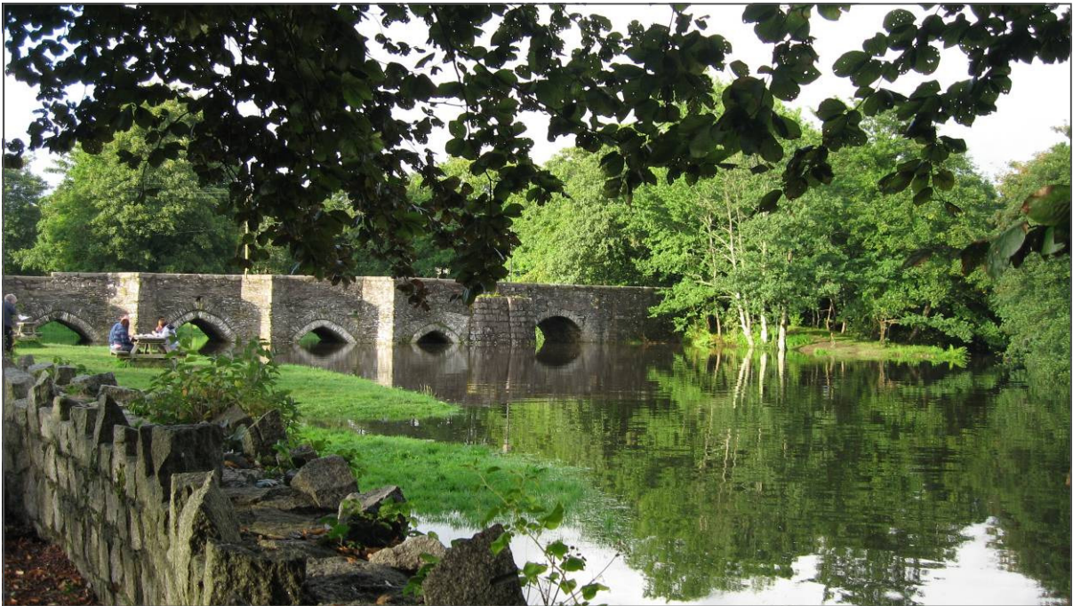
Lostwithiel Bridge at High Spring Tide
